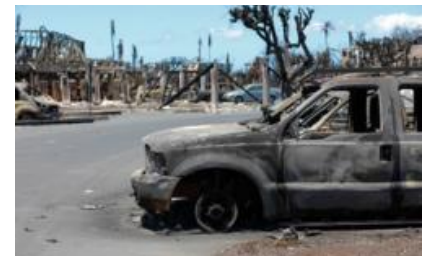
Damaged buildings and vehicles in Lahaina. [Sp. Sean Walker, photo.]
