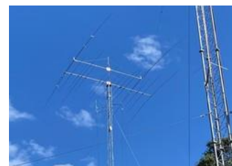
Tower 1 of the Tampa Amateur Radio Club, with the Force 12 C31XR antenna, second from the top. [Lu Romero, W4LT, photo.]
