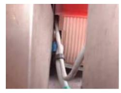
Here is a close—up of the cable entrance. There is just enough clearance to prevent the cables from getting crimped.
